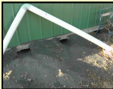
↑ Under concrete slabs.
