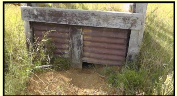
↑ In loading ramps.
