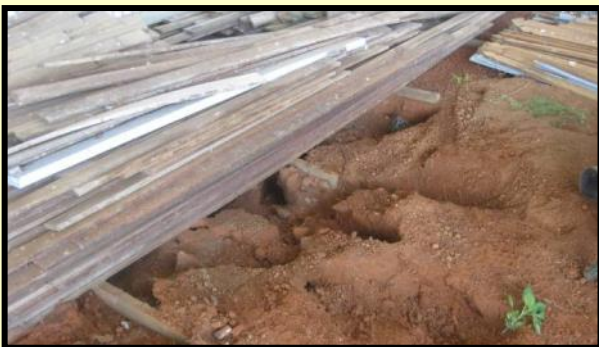
↑ Under materials stored on the ground.
