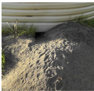
Water tank undermined by rabbits
