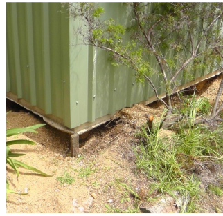
Concrete slab undermined by rabbits
